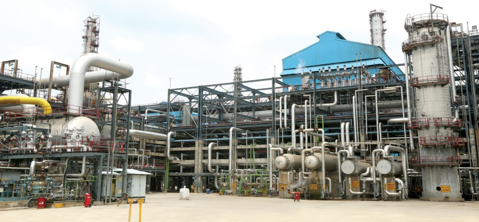
GAIL Pata Petrochemicals Plant
