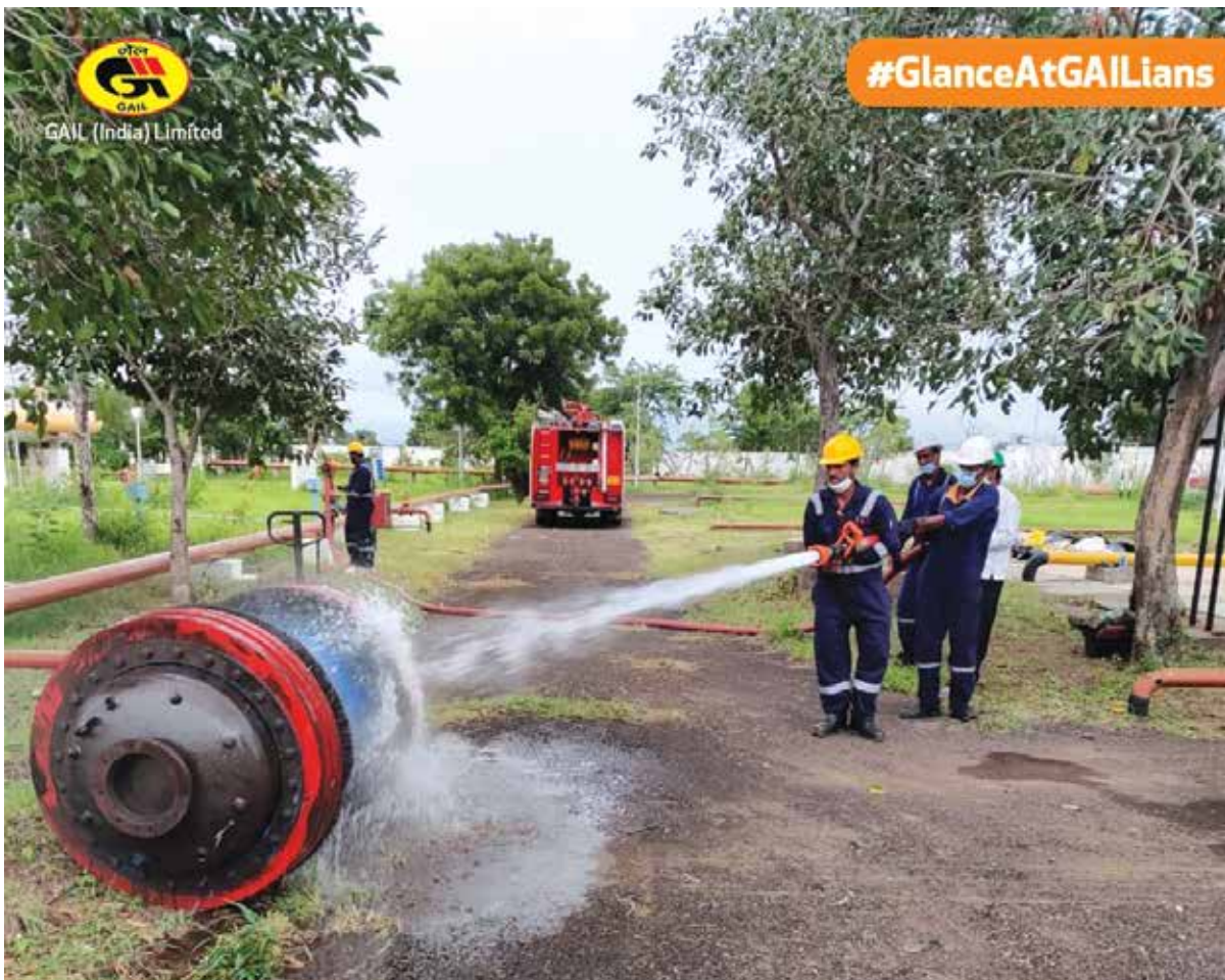
→ Operations and Maintenance (O&M) work at GAIL Khera, Madhya Pradesh
