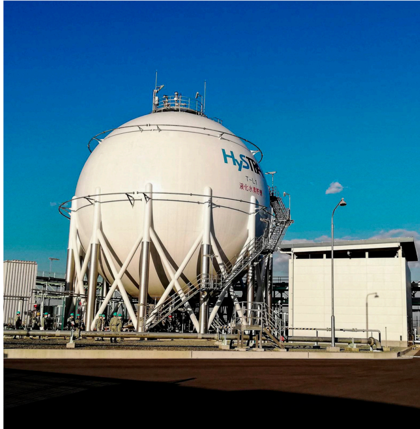
Scouting for more: A 2,500 cubic-metre tank containing liquid hydrogen at Kobe Port Island plant in Kobe, Hyogo Prefecture, Japan. AFP
