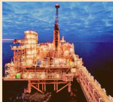
Covering 2.6 mn acres, the Mozambique Rovuma Area-1 Offshore project will entail development of integrated gas fields
